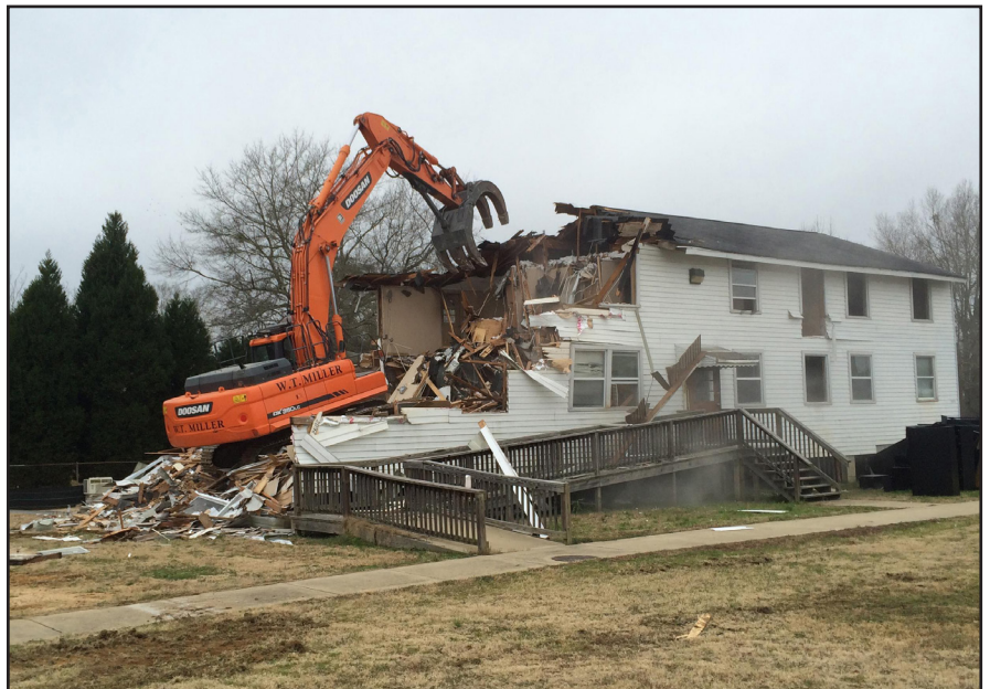
Soldiers Plaza, Bldg. 2602, a World War II wood building used most recently as an administrative facility, is demolished at Fort Benning, Georgia, under the Facilities Reduction Program.
